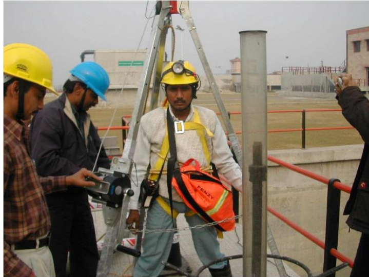
Typical Man entry with safety equipments
